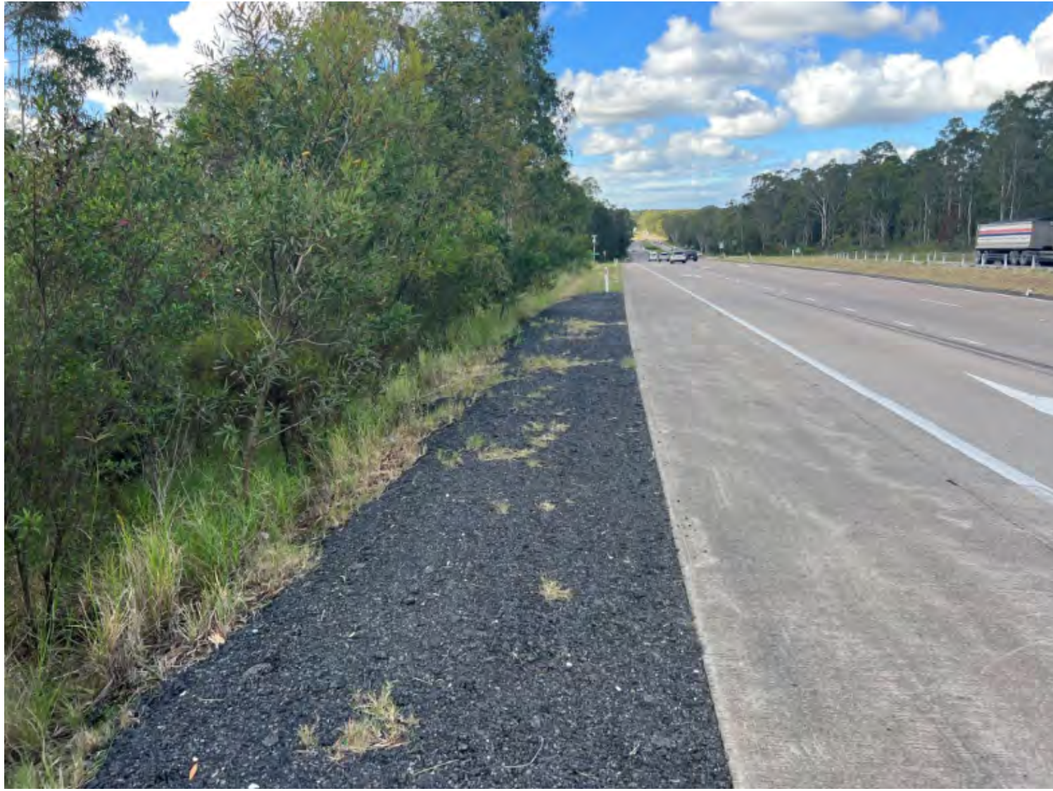
Photo 5 - Verge material (TfNSW R44 pavement material) north of Italia Road towards Balickera Canal
