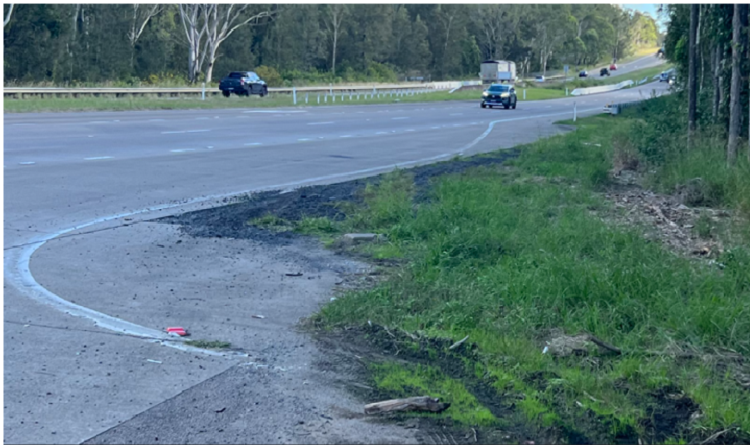
Photo 7 – Verge (TfNSW R44 pavement material) northbound approach to HWC access north of Balickera Canal.
