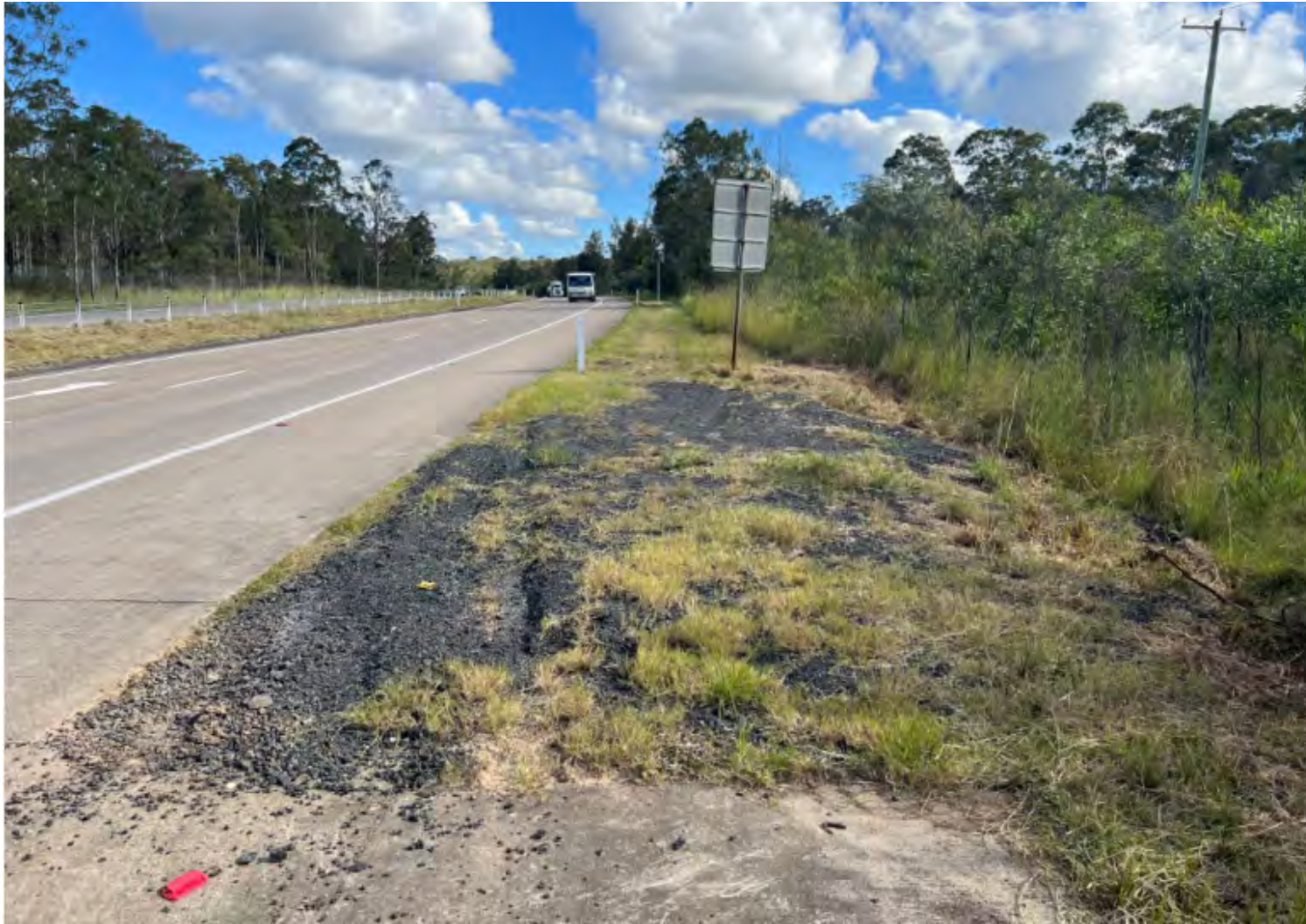
Photo 4 - Verge material (TfNSW R44 pavement material south of Italia Road (northbound approach to Italia Road)
