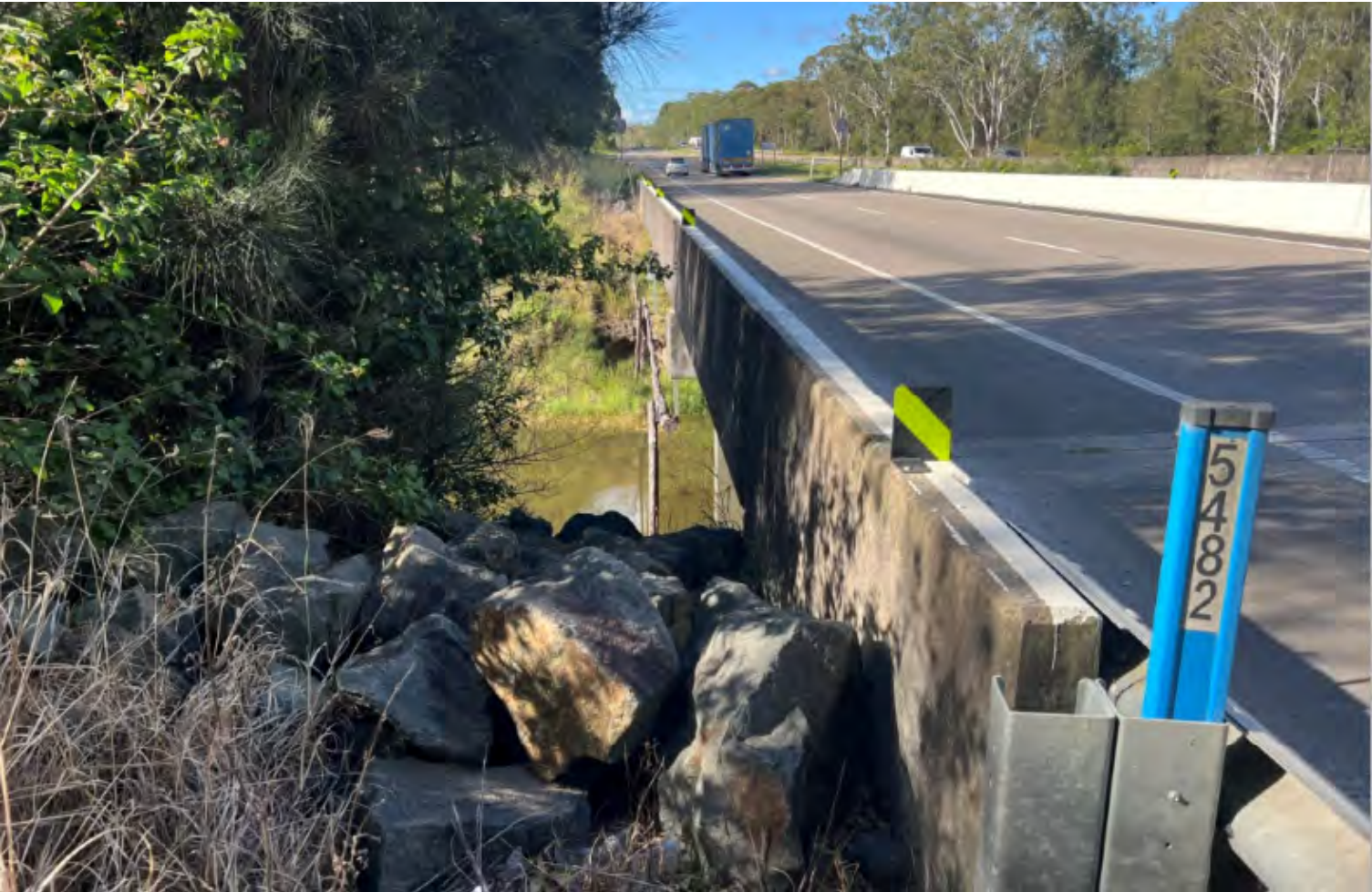
Photo 8 – Rock armouring of south-western embankment of Balickera Canal (northbound lane)
